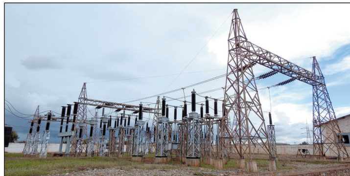
Sotrafer - 1x17.5 MVA, 120/11KV Switchyard
