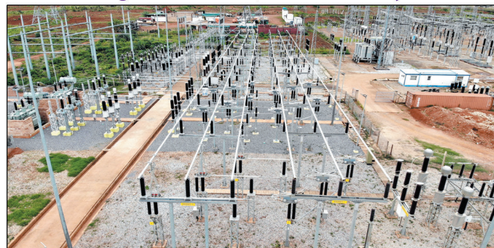
Fungurume - 2x5MVA,120/11 KV Switchyard
